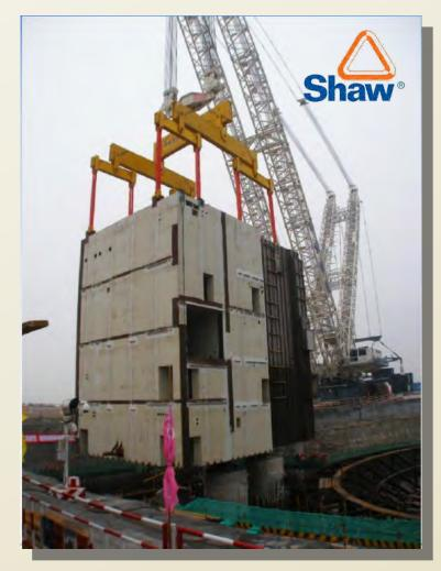
AP1000 reactor auxiliary building (China installation) same size as entire EM<sup>2</sup> module pair
