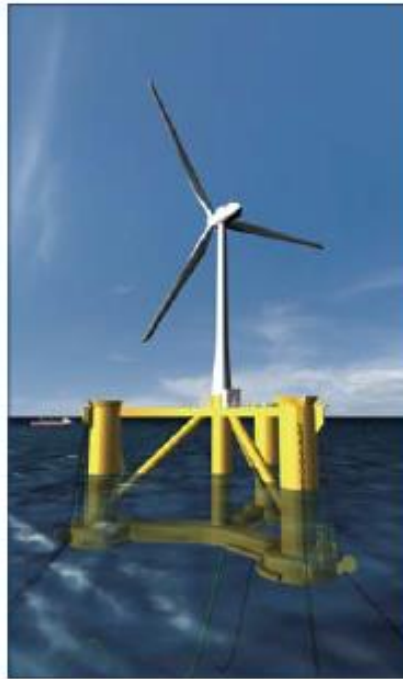
Compact semi-sub (WTG 2MW) 2013
