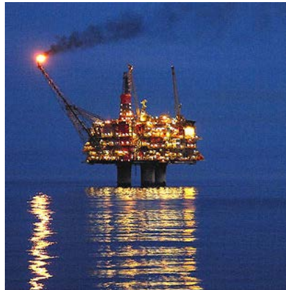
Subsea Oil and Gas
