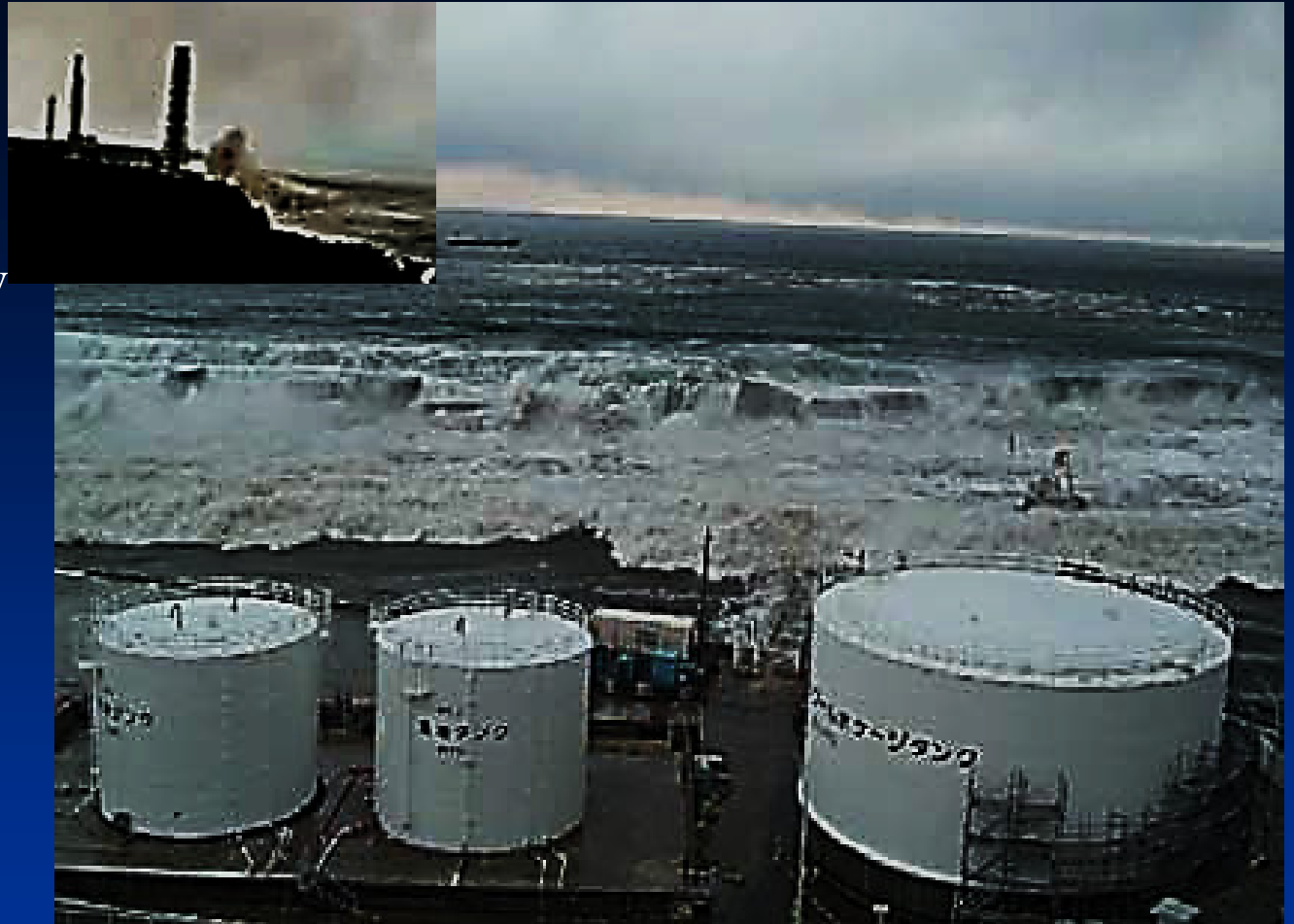
Tsunamis Attacking Fukushima Daiichi Nuclear Power Plant (Source: TEPCO)
