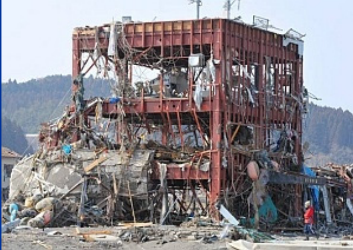
Disaster Management Center, Minami Sanriku, Miyagi, (Source: Kyodo)
