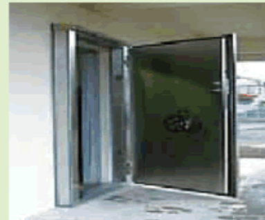
扉は水密扉へ取替
