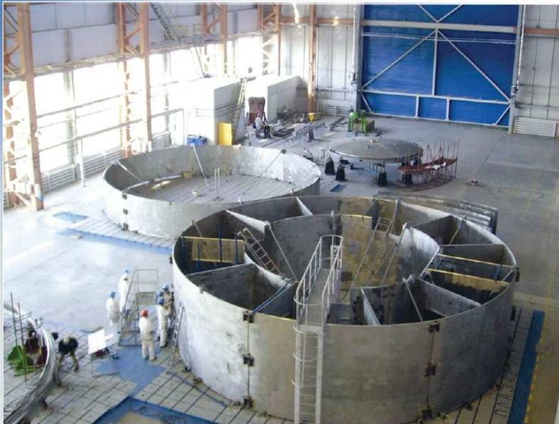
Installation of the reactor vessel bottom
