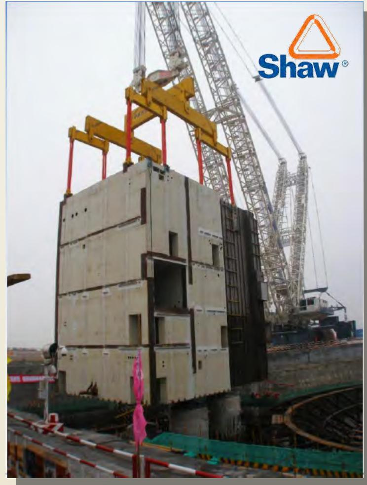
AP1000 reactor auxiliary building (China installation) same size as entire EM<sup>2</sup> module pair
